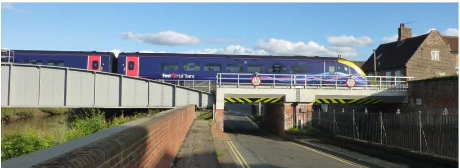
A Hull Trains class 180 unit crossing the low bridge at Selby. See page 8
