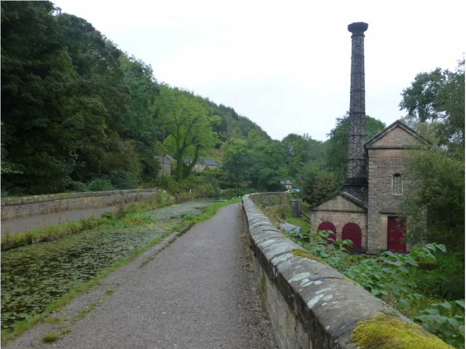
Leawood Pump House 26 September 2016.
