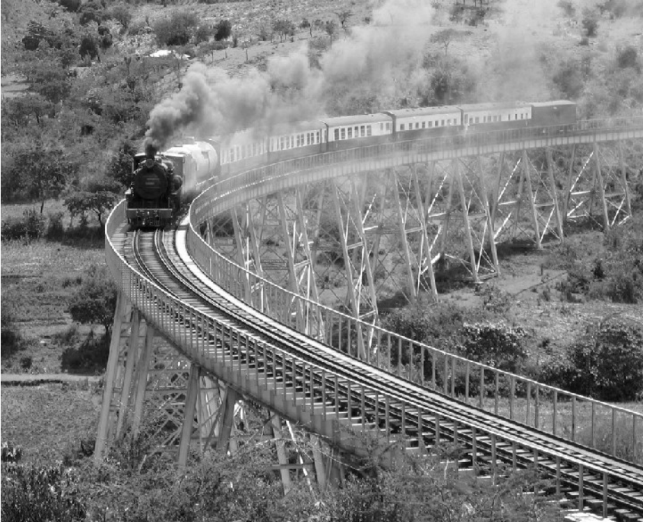
Crossing a steel viaduct.
