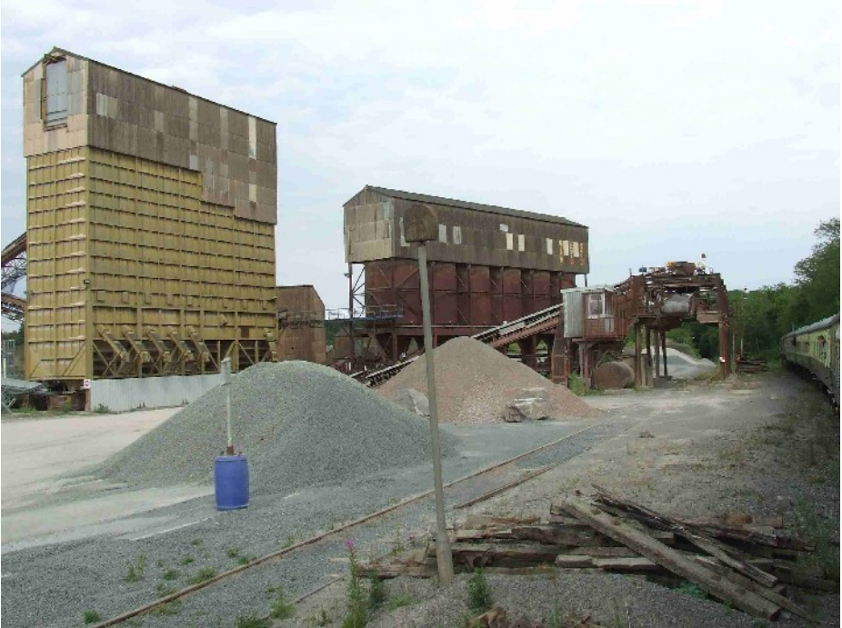
Tytherington Quarry loading area, with 66050 waiting to return us south.
