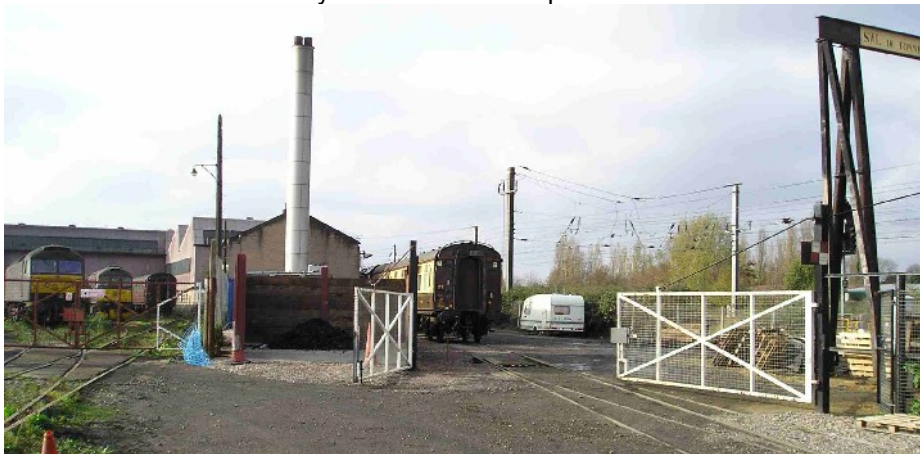
Locomotive Services on right (through white gates)
