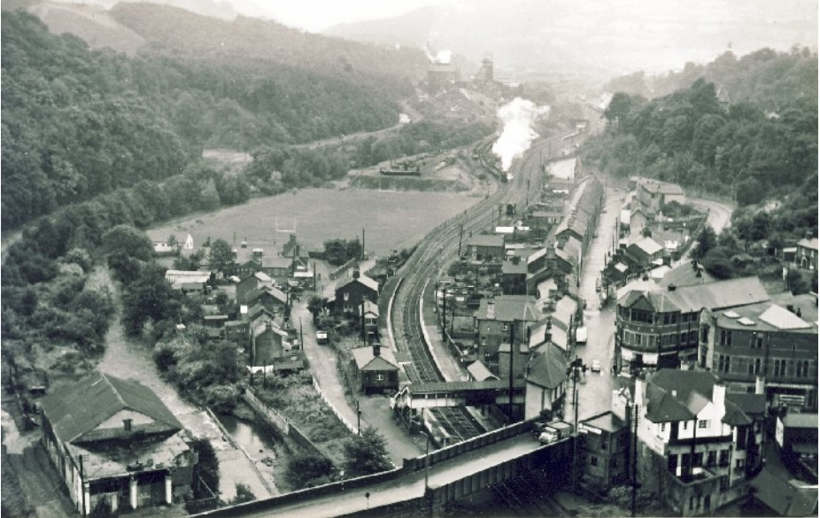
Looking south from a train crossing Crumlin Viaduct on 16 September 1960 showing Crumlin Station. In the distance a coal train pulls out of Celynen North Colliery probably taking a load of coal up to the Ebbw Vale steelworks. WRS A57
