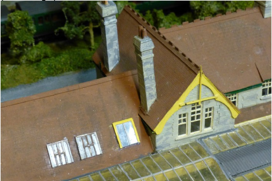
Photo 6 The restored chimney, the left hand one of the three; and the rooflights catching the 'sun' in this view.
