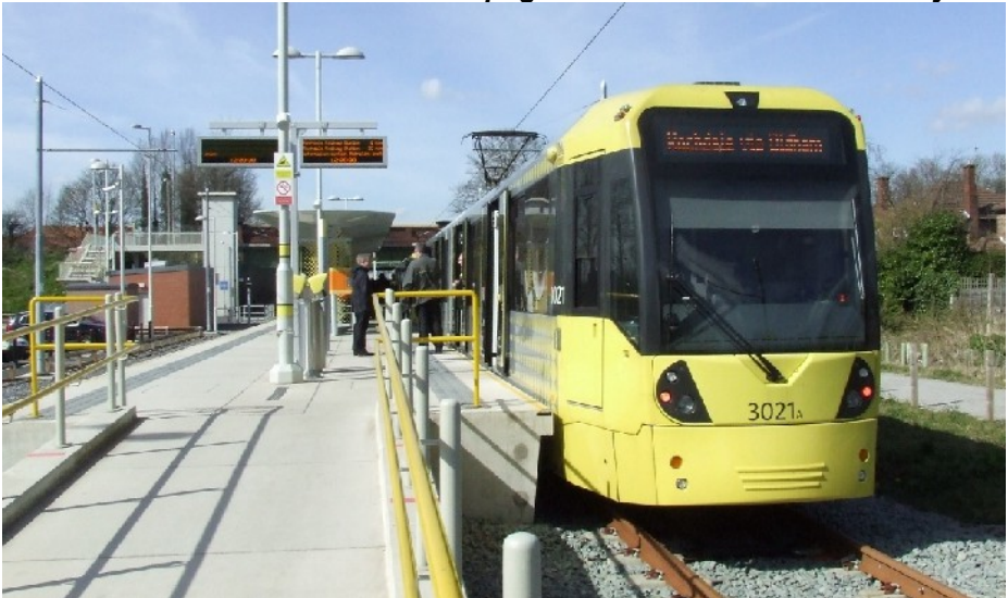
The other new tram extension is from St Werbergh's Road to East Didsbury where the terminus is on an old railway formation that continues behind the camera as a footpath. Ken Aveyard
