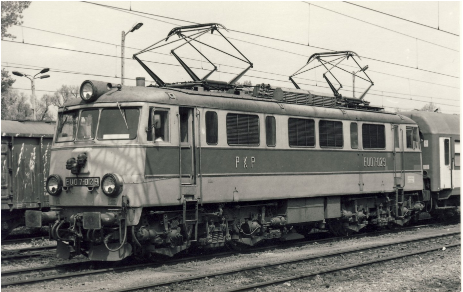
Polish Railways built class EU07 loco EU07-029 at Chabowka on 8 th June 1994. These were derived from the English Electric built class EU06 locomotives. WRS archive
