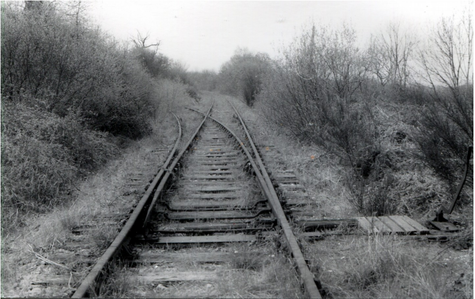
Carters siding at Corfe Mullen. The clay pit siding is to the left with the original line to Wimborne on the right. 24 April 1965. Colin Caddy
