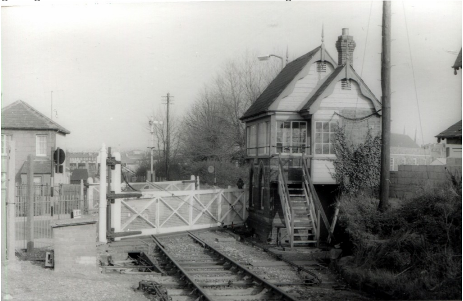
Littlefield Crossing Westham 11 February 1965.
