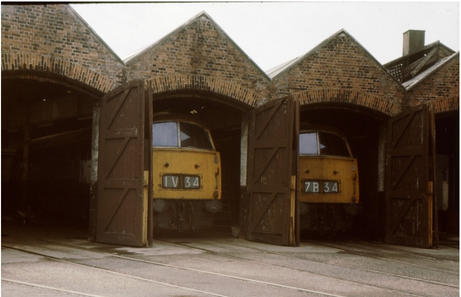
D1021 and D1033 are seen in the roundhouse at St Blazey 8 August 1975
