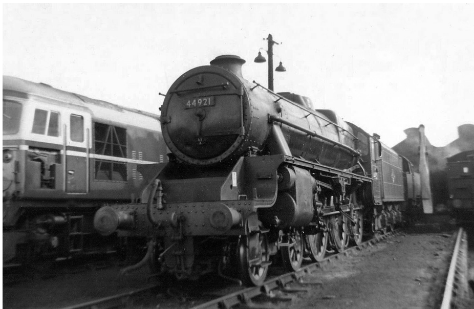
The mainstay of the Highland line in BR steam days were the Stanier Black Five 4-6-0's. 44921 is seen in pristine condition at 63A Perth MPD, June 1962. Worthy of note is the adjacent class 26, with automatic tablet catcher. See David Coasby article from page 5. Photo:Mike Brocklebank.
